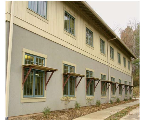
*Light shelves reflect sunlight onto interior ceilings to illuminate the offices without glare.*
