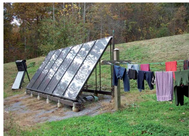
*Behind the dorm, solar panels preheat water to be piped inside for further heating by high-efficiency boilers.*
