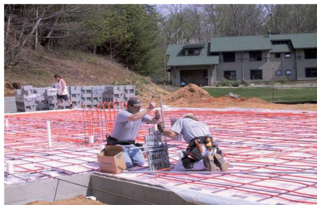
*Workers install the hydromatic (radiant hot water) floor heat system. The water is preheated in a solar collector, reducing the energy cost by half.*
